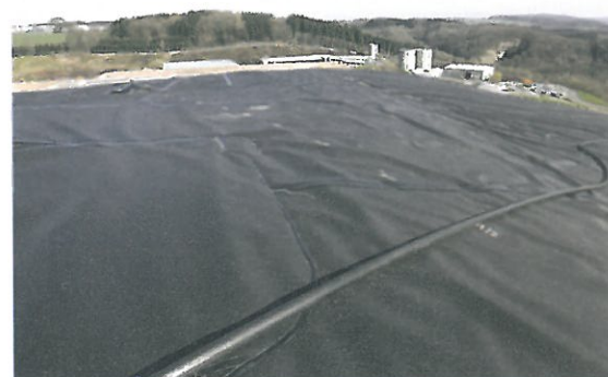
E A plastic sheet is used to help stop gases escaping from a landfill site.
