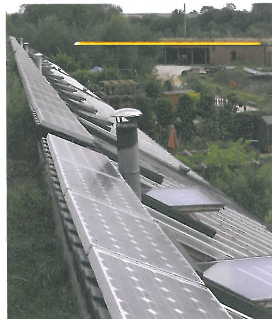
D The solar cells on the roof of the houses at Hockerton provide electricity for the people who live there.
