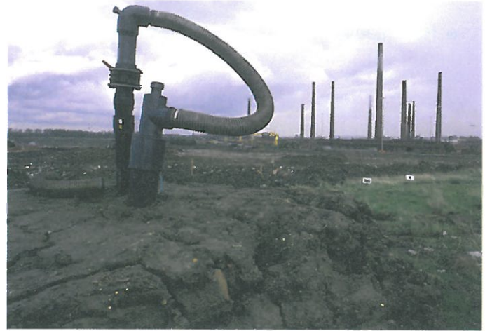
A These cracks were caused by gas collecting inside the landfill.
