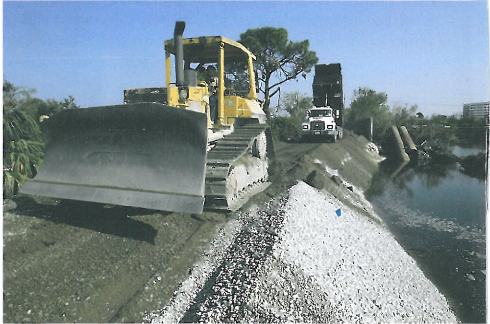
A This bulldozer is rebuilding a levee in New Orleans to prevent further flooding.
