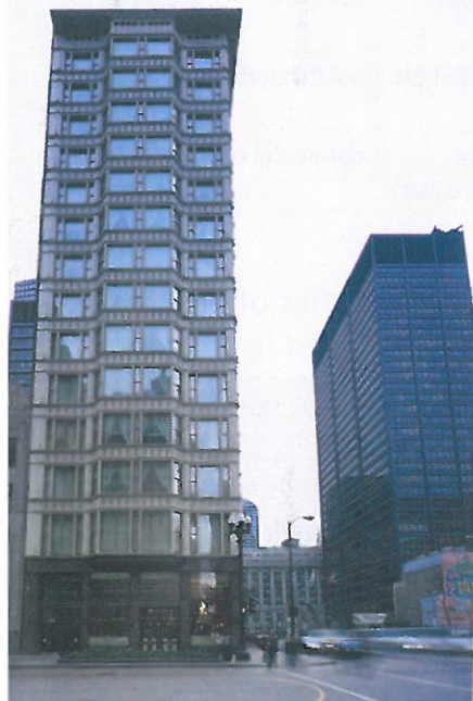
B The Reliance Building was built in 1895 in Chicago. It was one of the first large buildings to have a steel frame.
