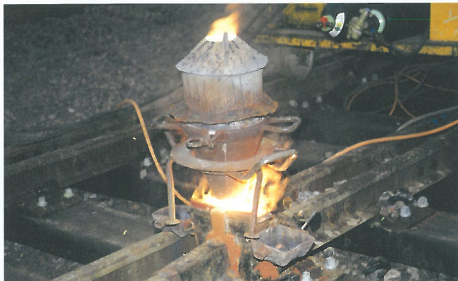
B The 'thermit reaction' produces molten iron.
