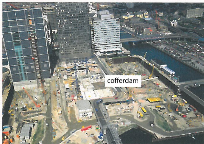
A Cofferdam keeping water out while the foundations for new buildings are constructed.
