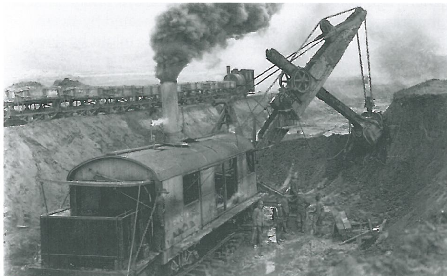
A Moving earth for dams or railway cuttings is much easier and faster with the help of machines. This steam-powered excavator was used to build a railway in the USA in 1906. It used levers and pulleys to move the digging bucket. Modern excavators use liquids to move digging buckets.
