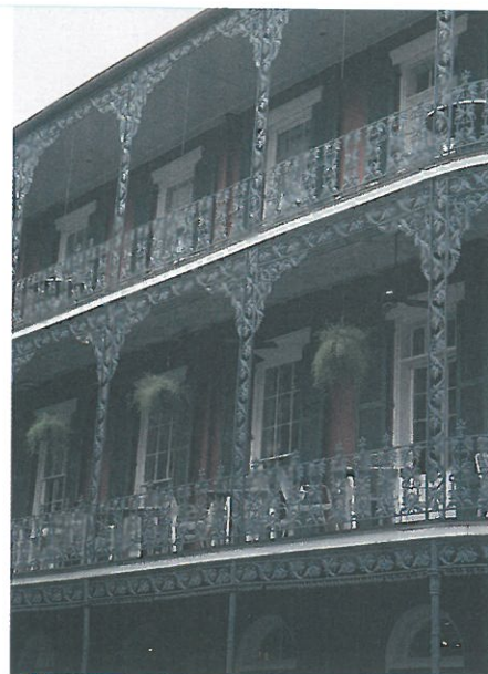
D These balconies are made from cast iron.
