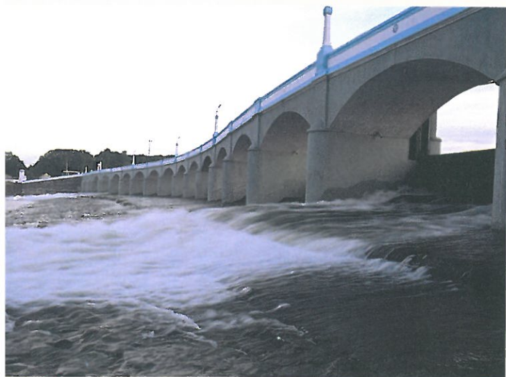
A A modern bridge built across the Grand Anicut (or Kallanai) dam, in Tamil Nadu, India. This is one of the oldest dams still in use. It was constructed from stone about 1900 years ago, to divert waters from the Cauvery river to use for irrigation.
