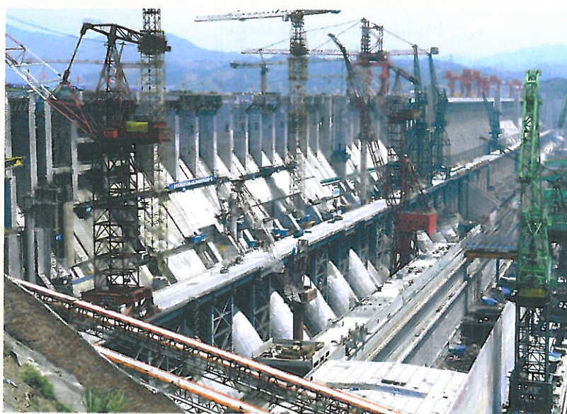
B The Three Gorges Dam, in China, under construction. When it is fully operational it will be the world's largest hydroelectricity power station, producing over 18 000 MW of electricity. It will also help to control flooding on the Yangtze River.
