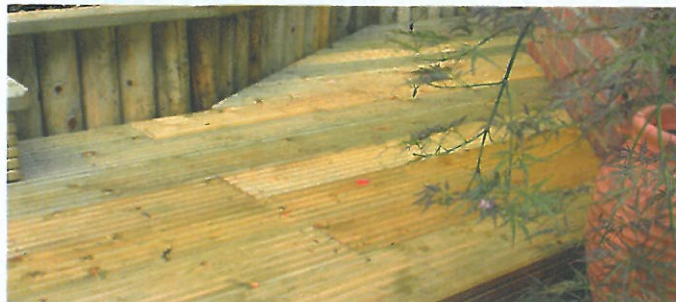
A Natural building materials can be treated with copper compounds to stop decay.
