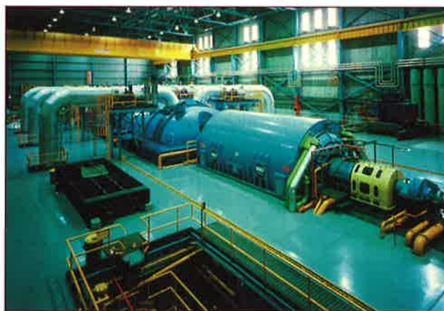
Figure 21.3 The turbine and generator in the generating hall of a Canadian nuclear power station. At the back are the turbines, fed by high-pressure steam in pipes. The generator is in the centre.
