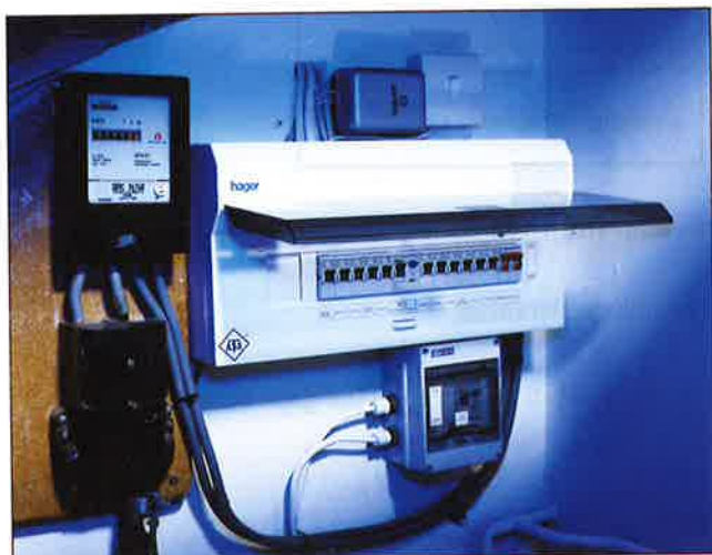
Figure 19.21 This is where the mains electricity supply enters a house. On the left is the meter. The white box contains a trip switch for each circuit in the house, together with an RCD, which protects the users of any circuit.
