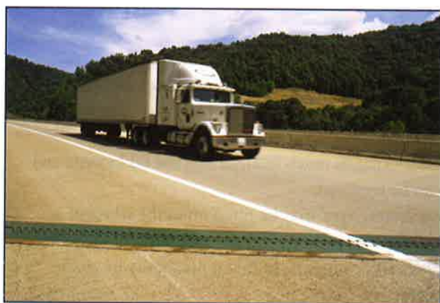
Figure 10.11 This truck is about to cross an expansion joint on a motorway bridge. On a hot day, the bridge expands and the interlocking 'teeth' of the joint move closer together.
