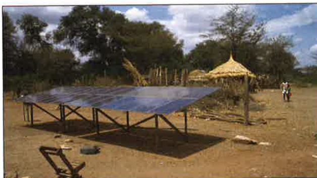
Figure 7.3 This array of solar cells provides electricity for a water pump in a Kenyan village.
